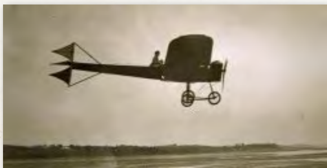
Harry in a Ferguson monoplane, Magilligan Sands circa 1911. Wingspan 32 ft, length 26ft, 8-cyl engine developing 35hp.
