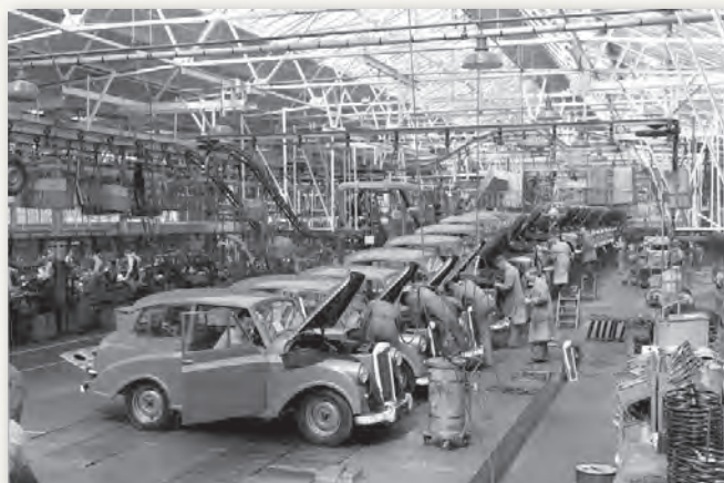
Mayflowers being finished on the line at Canley in 1951. Note that they are travelling 'sideways' as many models at Canley did in order to increase production rates.
